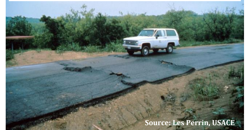
Heaving on Joe Pool Lake Road, Grand Prairie, Texas
