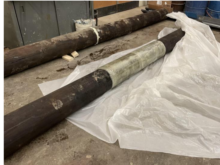
Completed FRP Splice
