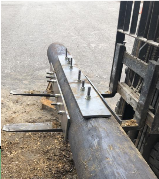
Completed Steel Plate Splice
