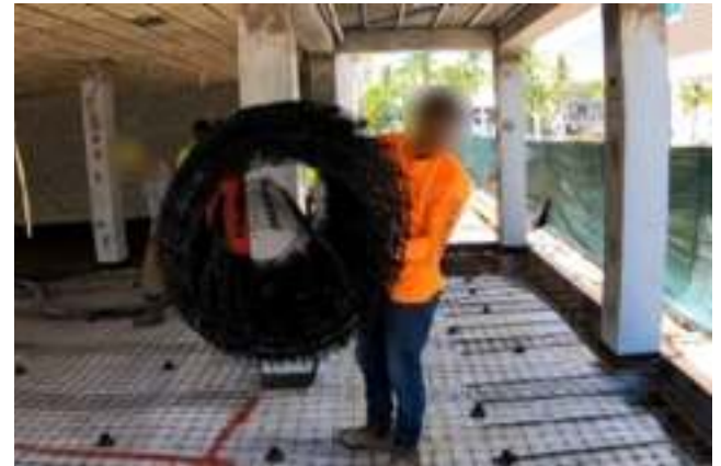
Fig. 5. GFRP mesh for slab-on-ground.
