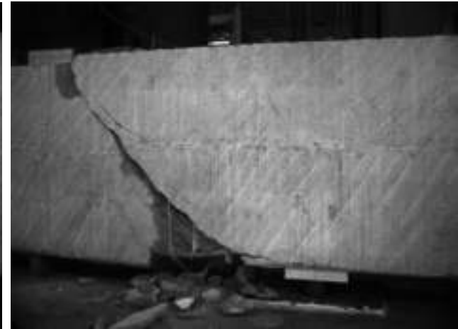
Failure Crushing of the top node and rupture of stirrups
