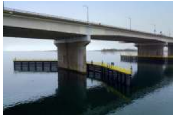
waterfront sheet piles
