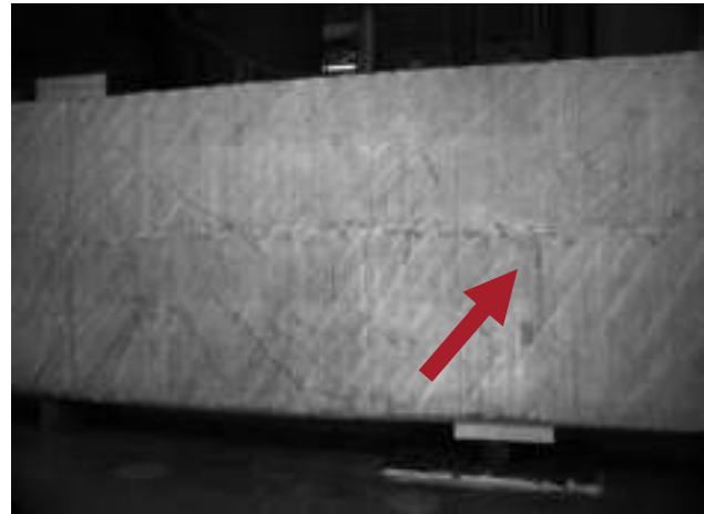
Peak Load Formation of a new diagonal crack
