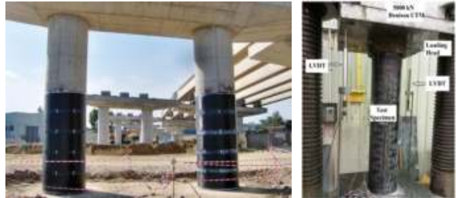
Fig.2. CFRP-wrapped Columns for bridge retrofitting 3,4 .
